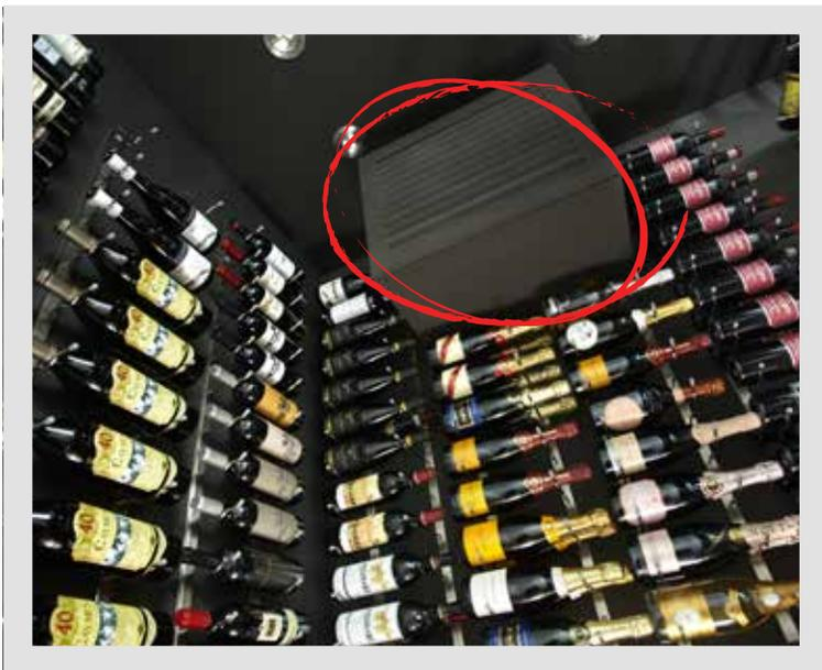
With this type of system, the unit is divided into two distinct blocks: the evaporator and the condenser. The evaporator is installed in the wine cellar, while the condenser is installed in an adjacent room or directly outside the building. The two components are interconnected by refrigeration lines. Must be installed by a HVAC specialist.
